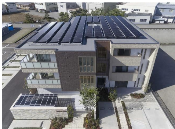
An example of Sha Maison ZEH rental housing construction
