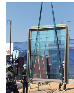
The SHAWOOD large-scale fixed sash combined construction method
