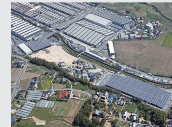
Yamaguchi Factory mega solar
