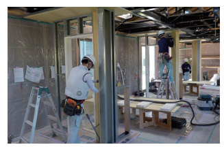
Interior finishing course: completion test
