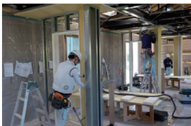
Internal construction test course
