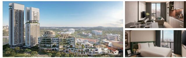
One Holland Village (Complex development business) Distant exterior view (left)/Interior (upper right and lower right)
